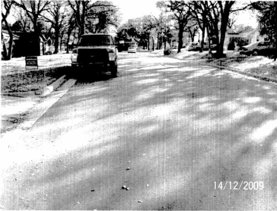
Picture #1-Roadbond en1 treated area-Near perfect condition.
