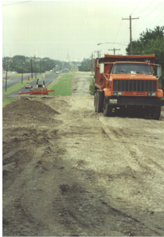
Dallas Military Pkwy, spreading base
