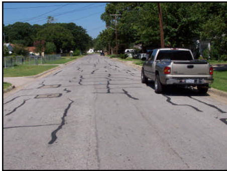
an asphalt overlay.
